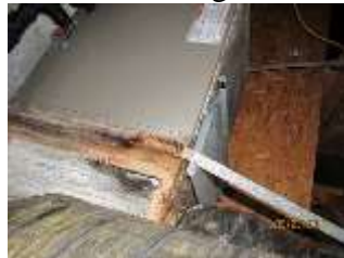
Above photos and photo below show damage done to a/c units from incoming water
