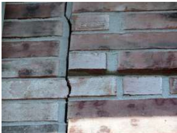
All photos on this page show cracks in and around the front overhead garage door area
