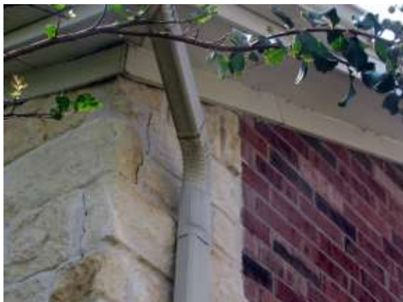
All photos on this page show cracks in and around the front overhead garage door area
