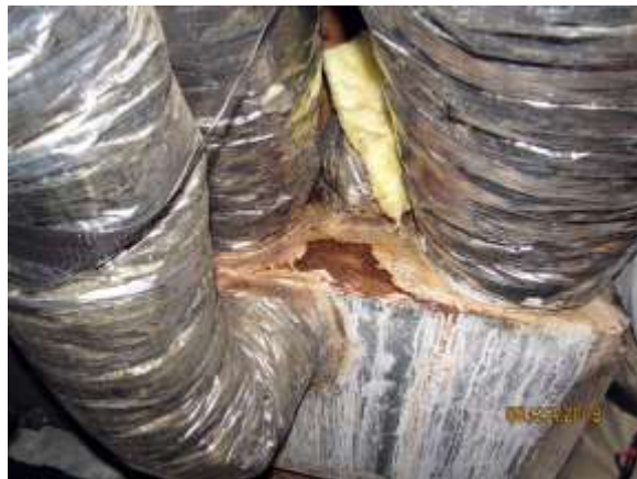
Above photos and photo below show damage done to a/c units from incoming water
