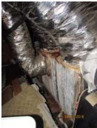
Above photos and photo below show damage done to a/c units from incoming water
