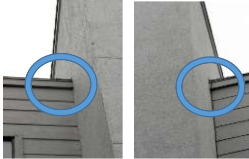
Locations where kickout flashing is required
