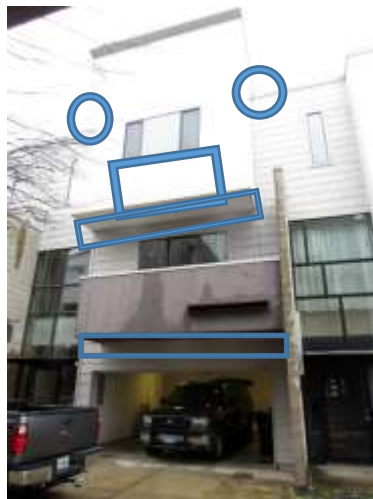
Areas outlined in blue show where stucco removal is needed
